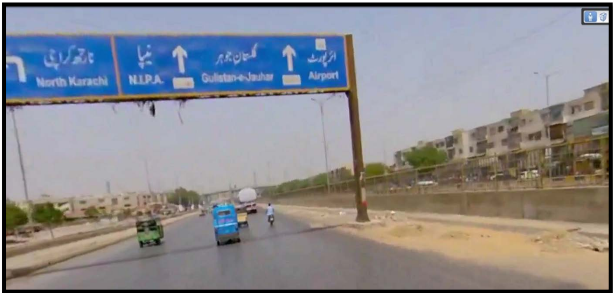
Figure 4 Pole in the fast lane before Nagan Chowrangi flyover.
